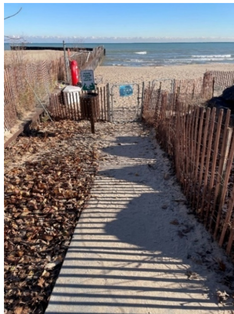
Figure 2-1. Existing north entrance concrete ramp, looking from the initial gate downward toward Lake Michigan.
